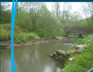
Weir removal River Medlock
